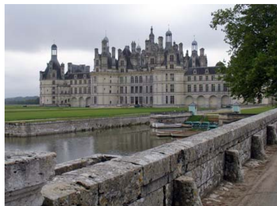
The famous Loire Valley Chateaux were built with the same tuffeau limestone that you can find in the soil of Vouvray.
